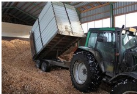
Figure 34. Unloading of chips to fuel storage (Alakangas, 2013)
